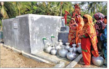
suitable option for drinking water. People drink the pond water without any purification. As a result, most of the inhabitants of salinity affected area suffer from different water borne diseases. Pond Sand Filter (PSF) in the salinity risk zones has been introduced to reduce the deficiency of safe drinking water. 53 ponds are re-excavated with PSF for ensuring safe drinking water for the targeted beneficiaries of salinity intruded areas.
