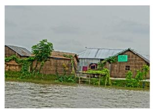
Figure 3: Raised plinth stands high above flood water
