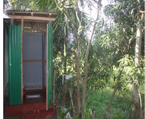
Figure 3 Neat and clean Sanitary Latrine
