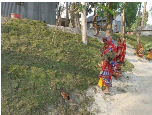
Photo 8 Turfing the grass in a cluster Uttar Borul under Islampur Upazila, Jamalpur: IE: SSS.
