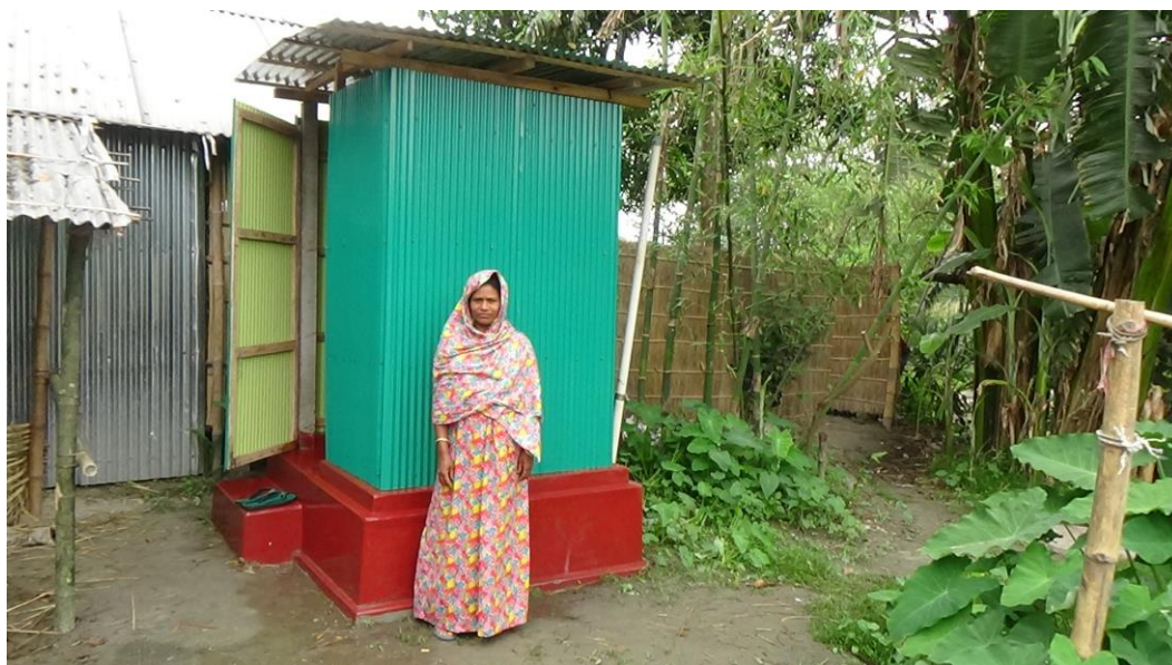
Photo 4 Construct of climate resilient sanitary latrine, Kurigram, IE:NDP
