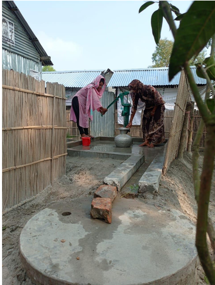
Photo 4 Installed Climate resilient Tubewell on raised Plinth, Kurigram: implemented by NDP
