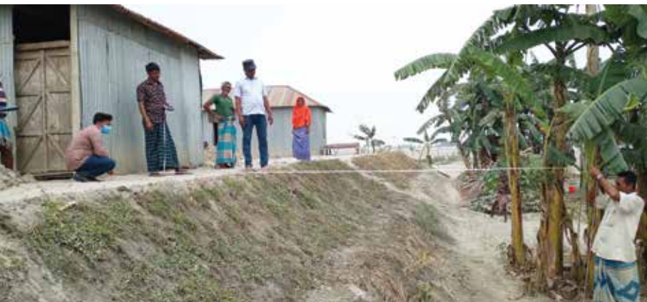
The height of Sabina's raised homestead plinth being checked
