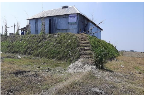
Figure 10-11: Turfing in the slope of the raised plinths
