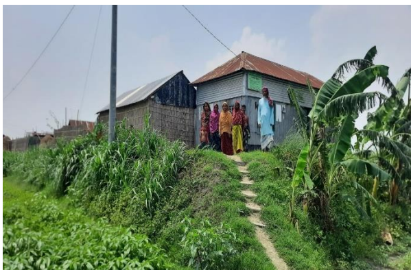
Figure 10-11: Turfing in the slope of the raised plinths
