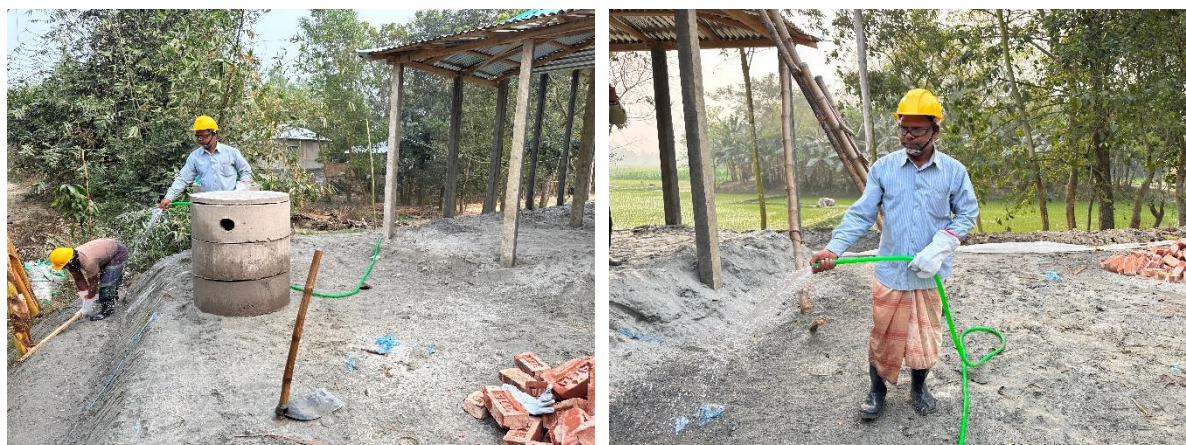
Figure 5.1: Water Sprinkling to Arrest Dust
