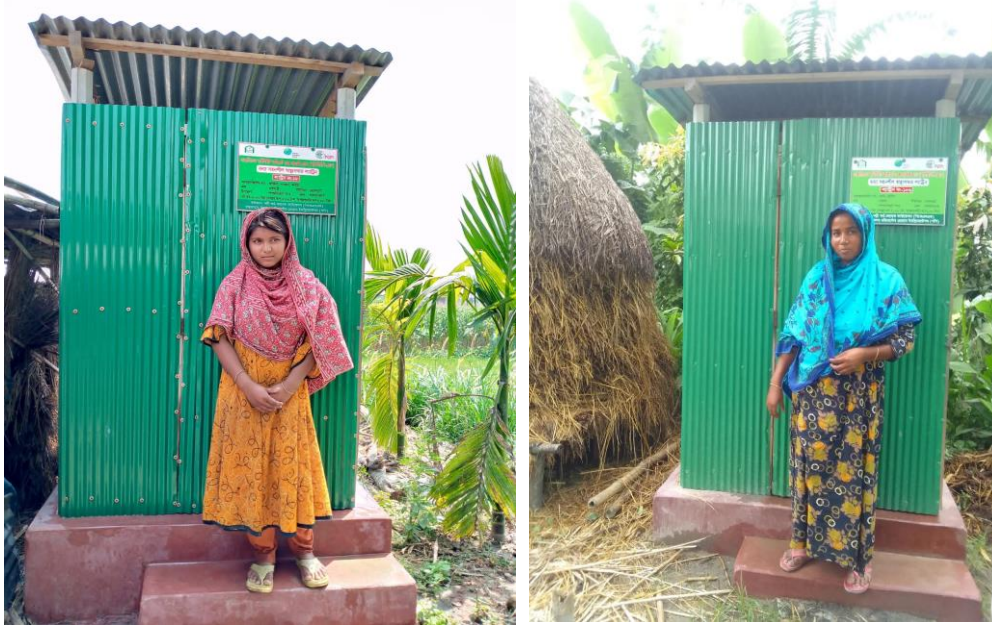
Photo 5: Construct climate-resilient sanitary latrines
