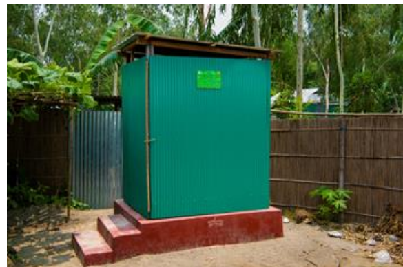
Figure 2: Flood resilient Sanitary Latrine
