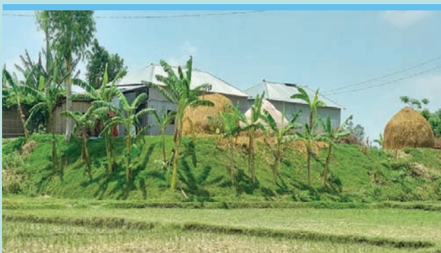
Cluster-based homestead plinth raised in Gaibandha
