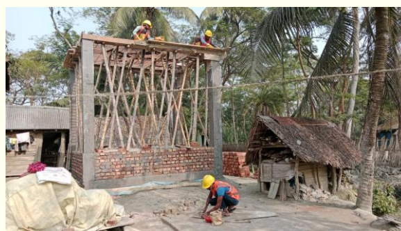
Construction work of disaster resilient house
