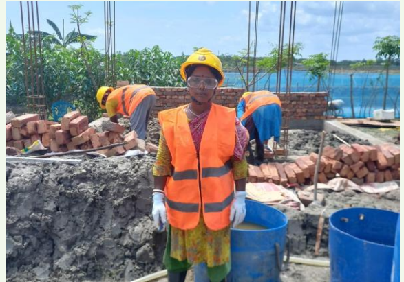
Eitika working at a climate-resilient homestead construction site
