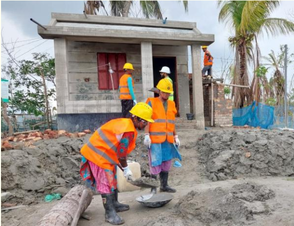
Construction of resilient homestead in progress
